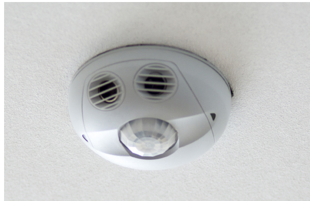
Lighting vacancy sensors save energy by turning off lights automatically when rooms are empty.
